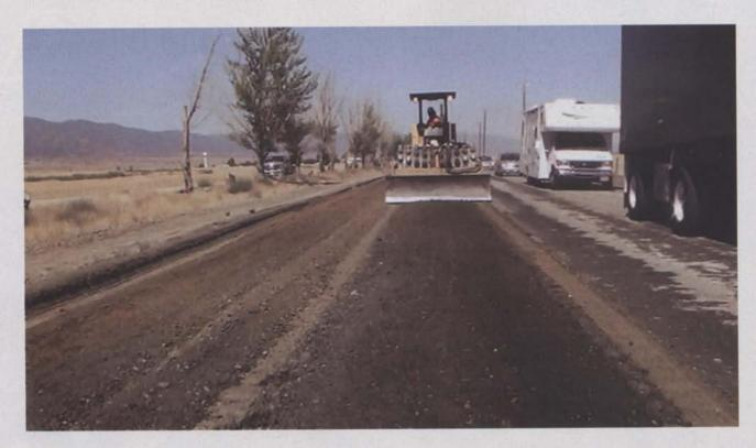
much thinner in areas that had been milled to correct the slope. And along the shoulder areas more oil was required in the recycling process to accommodate the widening Caltrans called for in adding a 4.5-foot paved shoulder to the 12.7-foot travel lanes.
