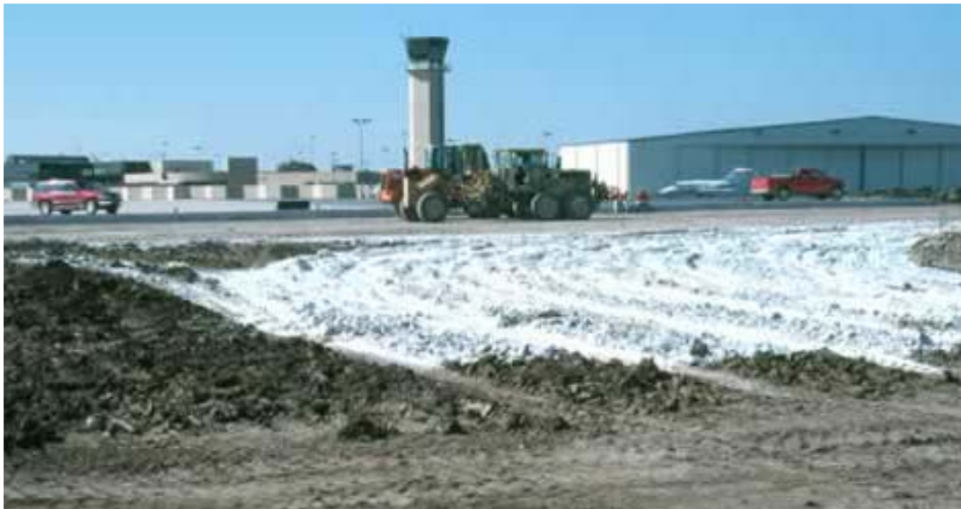
Figure 21: Lime stabilization project at an airport
