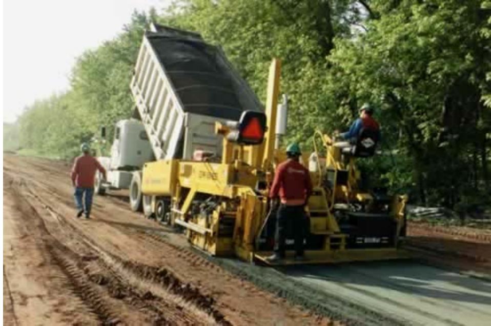
Figure 20: Asphalt paving machine used to spread moist fly ash
