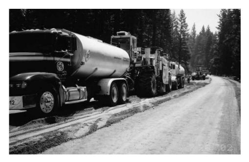
compacting, grading and finish-rolling. Aggregates may include pulverized material from the existing roadway, soils, additional processed or native aggregates, or additives such as cement or fly ash.
