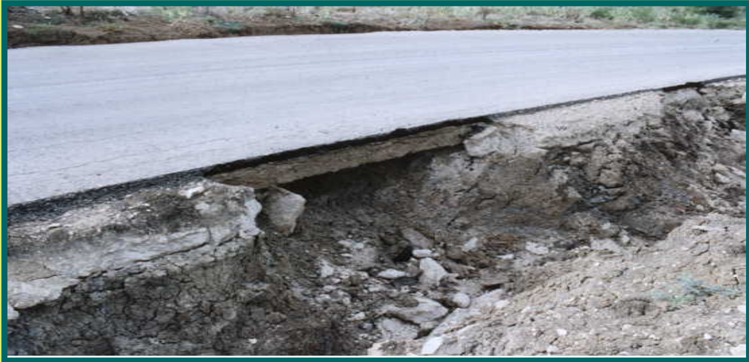
Lime subbase bridging an erosion failure
